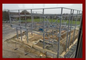
Good progress is being made on the new building with the steel frame now in place.
